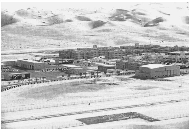
Fig. 7. Shaybah community surrounded by mega sand dunes; community is well protected using variety of protection systems, including system of sand drift fences
